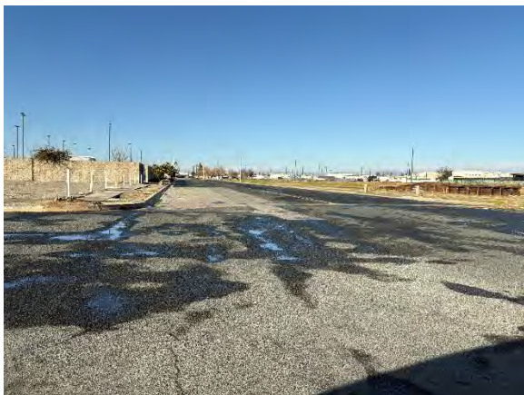
-Glenwood Street Facing North-
