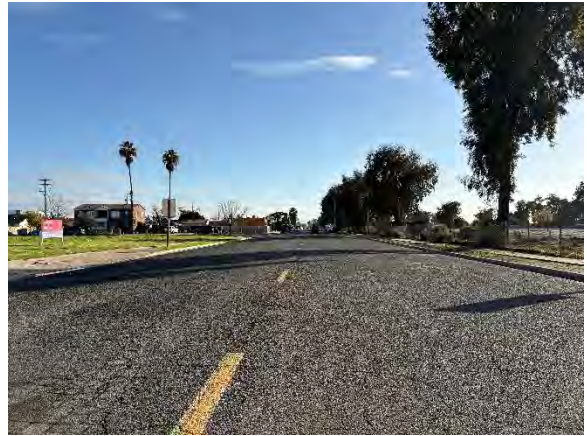
-Fremont Street Facing South-
