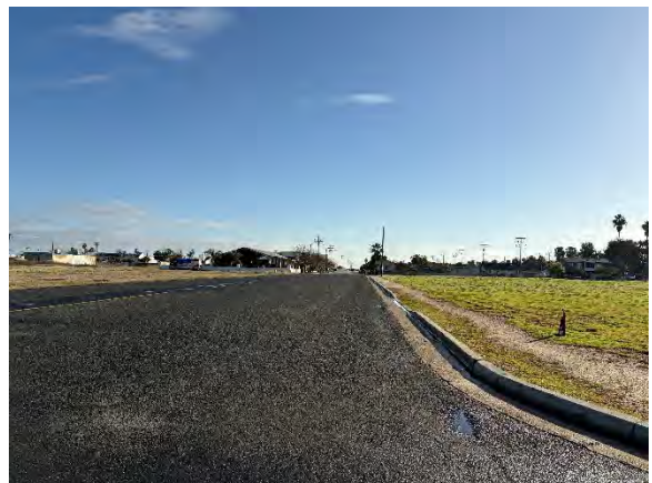
-Glenwood Street Facing South-
