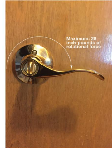
Operational force for door hardware.
