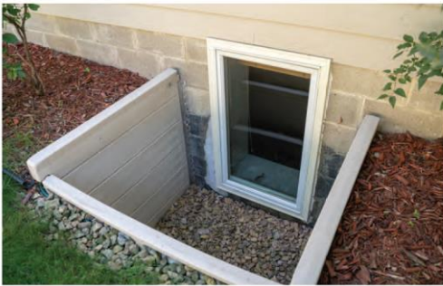
Typical emergency escape and rescue opening.
