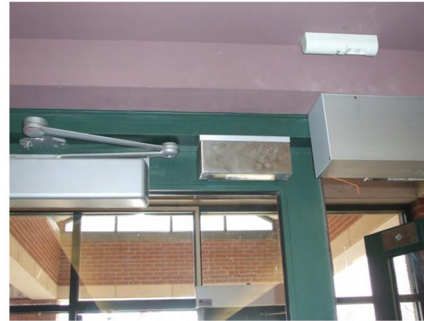
Door closer and electromagnetic lock projecting into door height.
