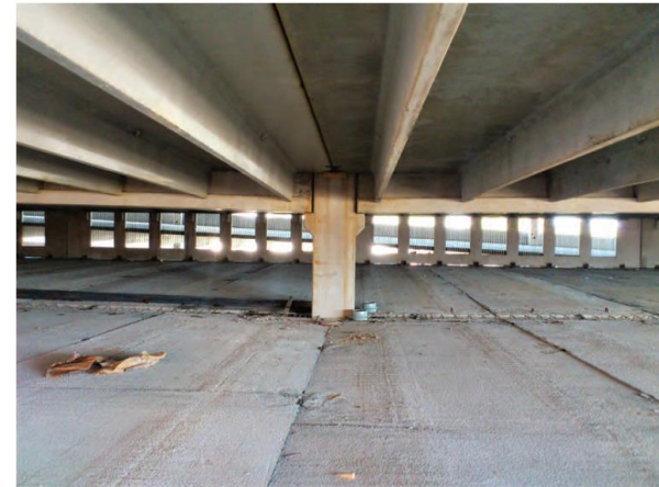
Precast concrete diaphragm construction.
