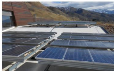
Examples of roof dead loads – HVAC equipment, solar panels and vegetative roofs.
