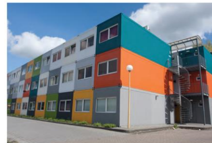
Multi-level structure of intermodal shipping containers.
